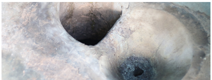
Image 2. EcoSan Toilet-Urine Diverting Front End
